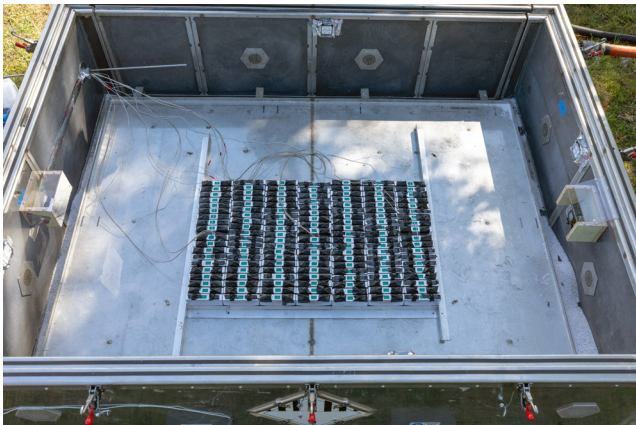
Test sample pre-test - batteries assembly installation
